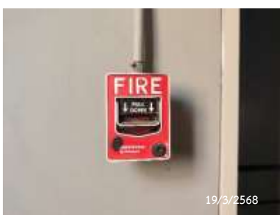
Fire Alarm Manual Station
