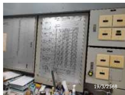
Graphic Annunciator Fire Alarm System
